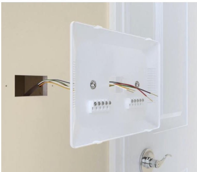
Figure-7: Remove Thermostat Face and Base Plate. Figure-8: Secure all unused Thermostat wires.
