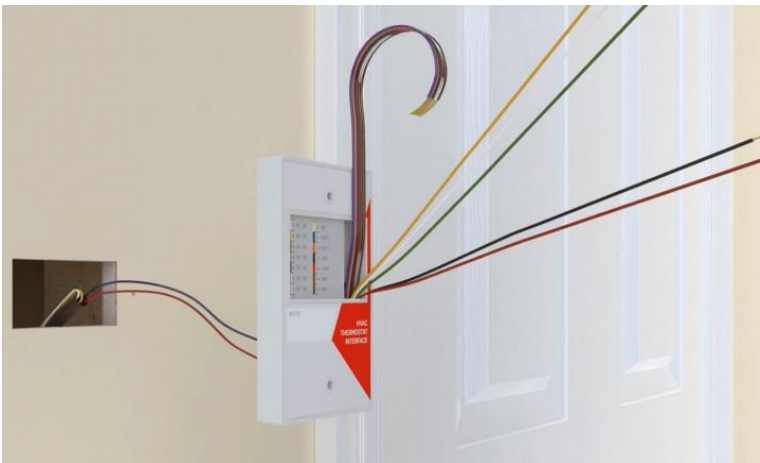
Figure-11: Feed the wires through the back of the Thermostat base plate and connect to the Thermostat terminal block.
